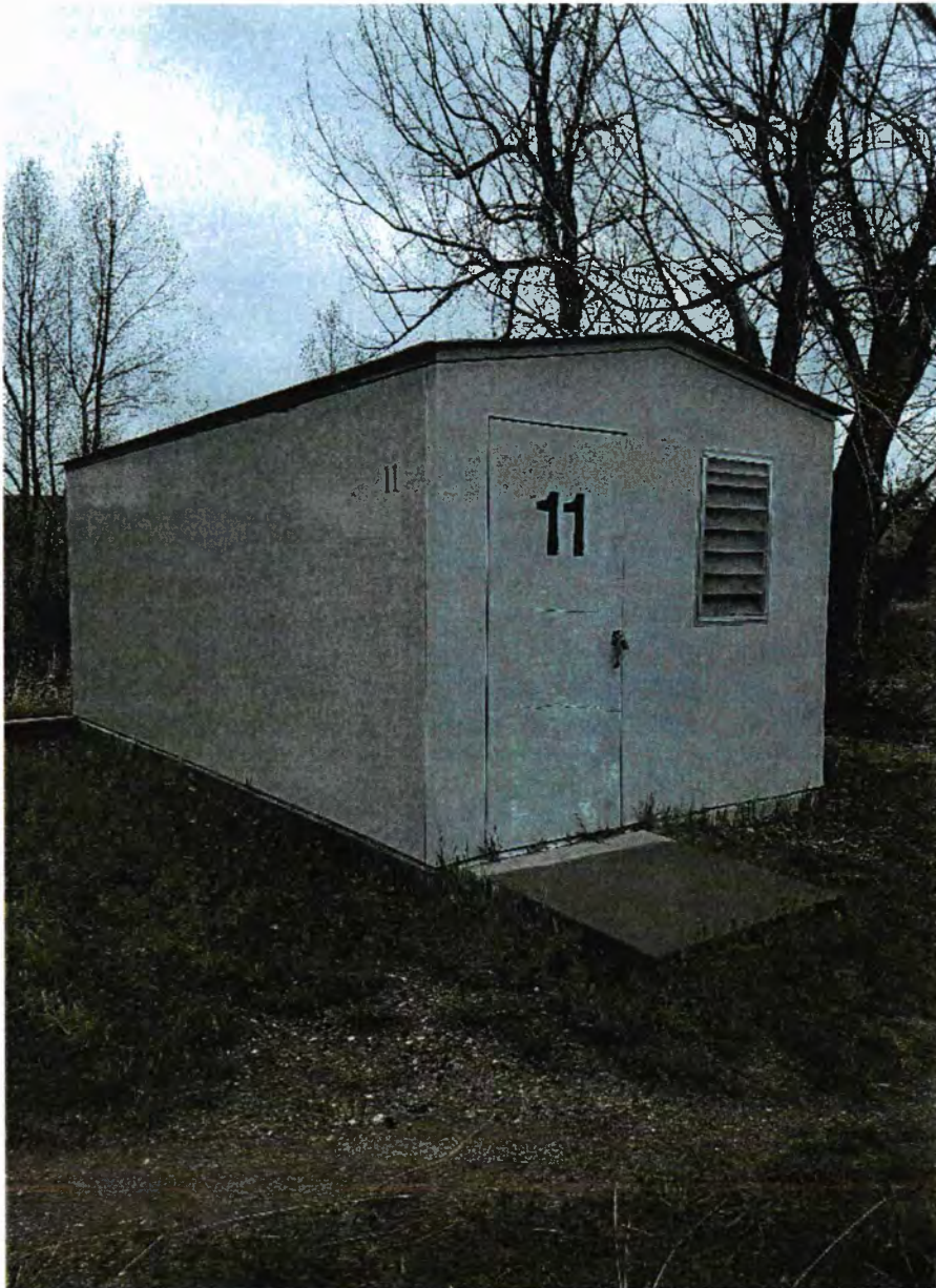
Water well number 11 located on the Property
