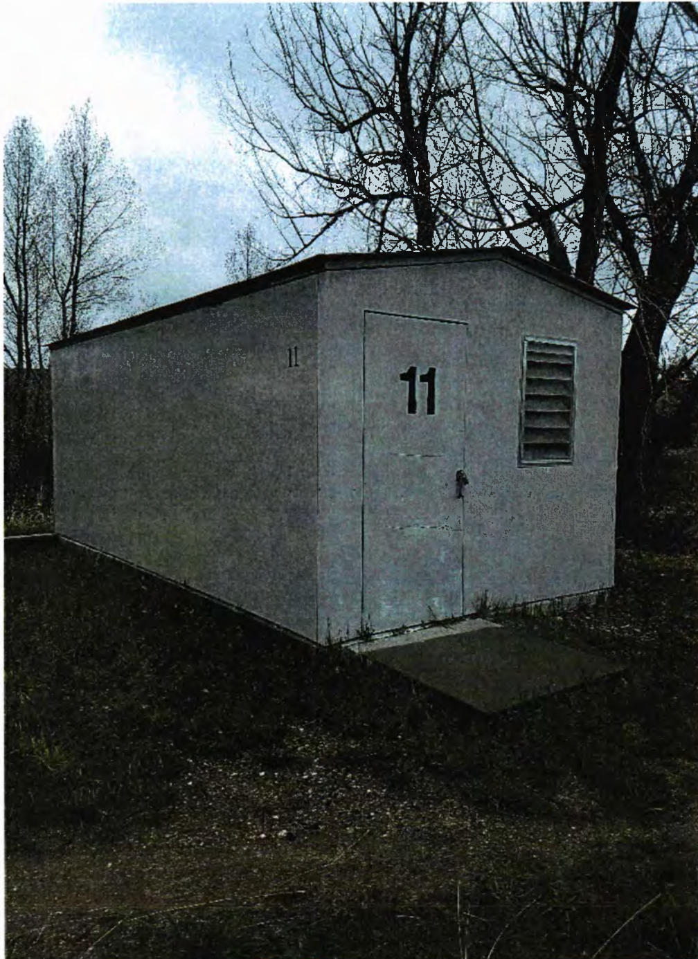
Water well number 11 located on the Property
